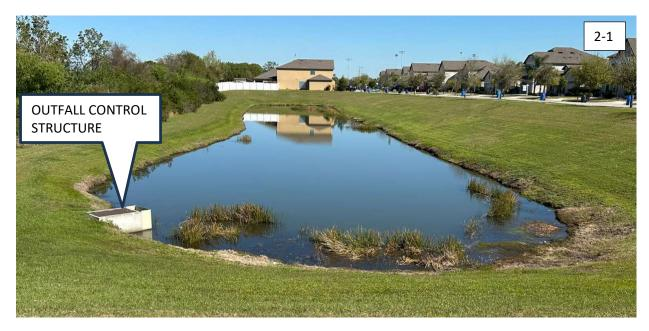
The concrete outfall control structure (lower left corner of photo 2-1 above) did not reveal any obvious deficiencies. Upon closer review, however, we believe that the bleeder device is obstructed since the water level in the pond is at the weir crest elevation and not at the invert elevation of the bleeder device (6" PVC tee). Therefore, the water elevation in the pond is too high (by approx. 1 foot). The bleeder device will need to be cleared of any obstructions by the aquatics contractor.
